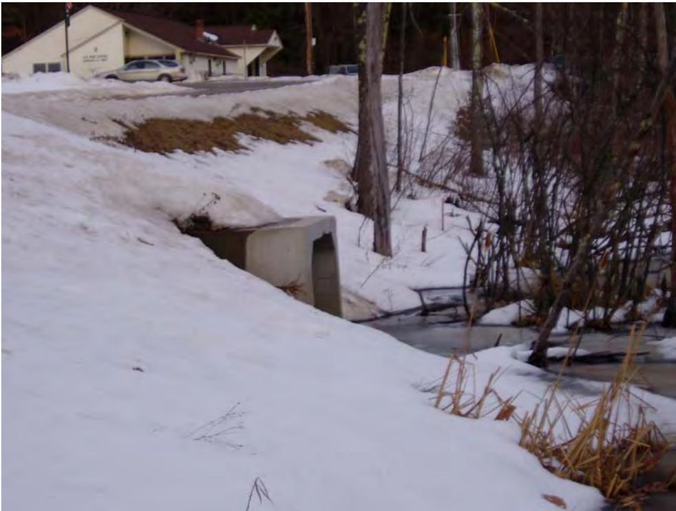
4. This photo shows the large 4' x 4' concrete culvert that connects the upper and lower reaches of Wetland #15. This existing culvert passes beneath Glastonbury Drive, the road that provides access to Avalon Estates.
