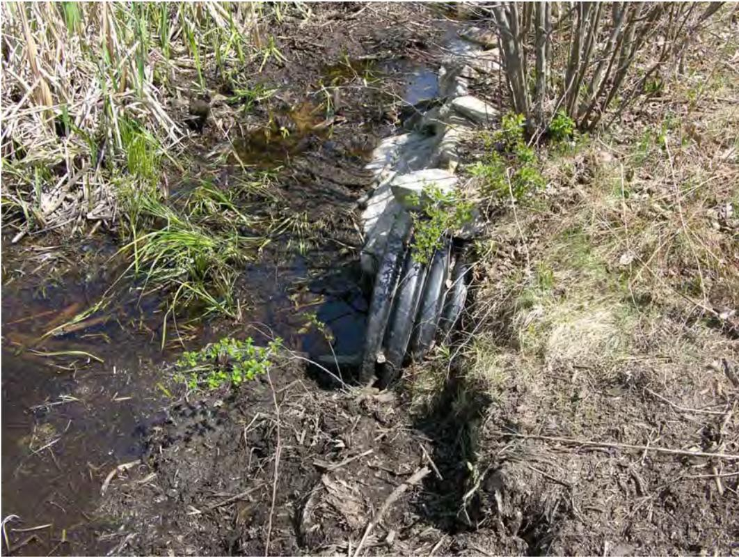
5. This is a view of one of the three 24" diameter culverts which connect Wetland #9b to #9a under the residential driveway.
